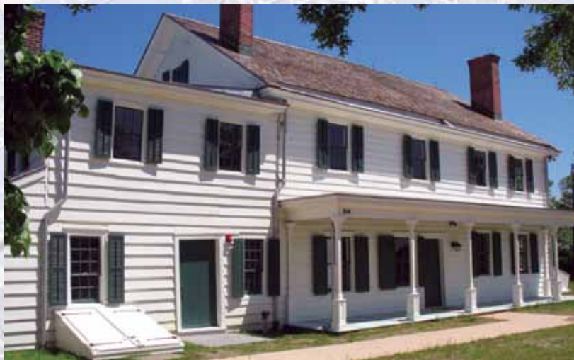
The renovated Bayshore Activity Center.
