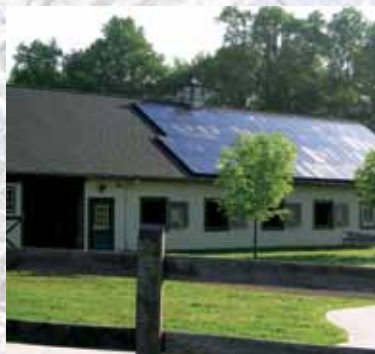
New solar panels at Sunnyside Equestrian Center.
