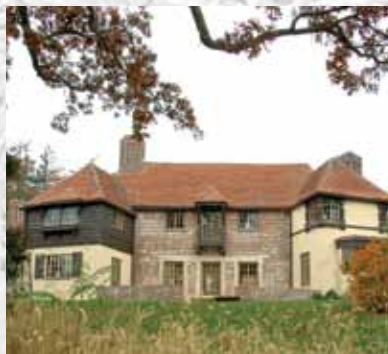
Exterior renovations at the Huber Woods Environmental Center
