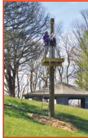
The Challenge Course at Big Brook Park was repaired and expanded.
