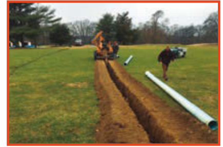
A new irrigation system was installed at Shark River Golf Course.
