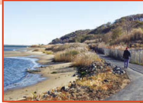
Waterfront sections of the HHT were stabilized prior to reopening.
