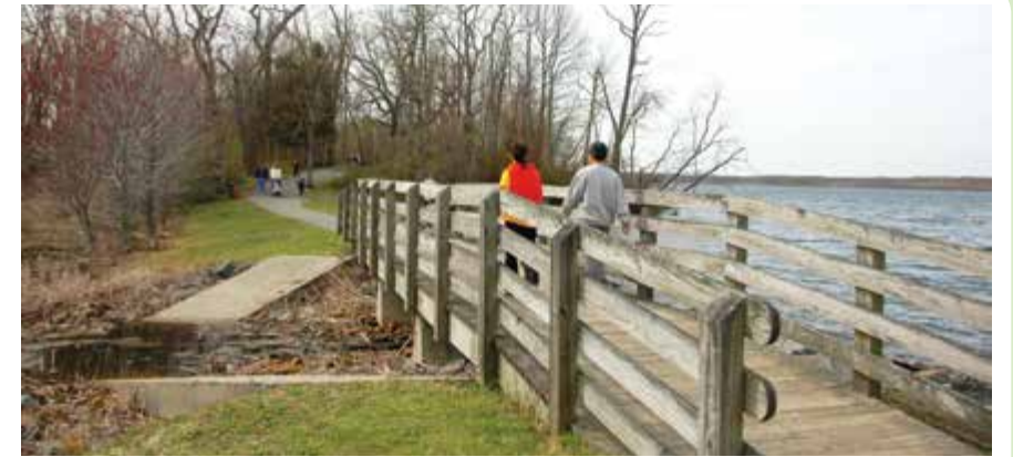
A bridge crossing over a wetland dike at the Manasquan Reservoir.
