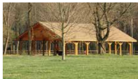
A new picnic shelter was constructed at Thompson Park.
