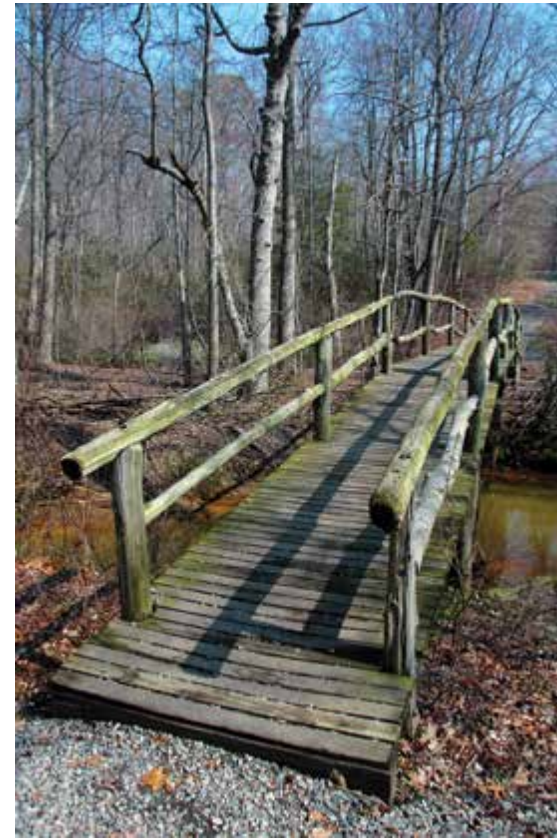
The first trail bridge, built in the early 1960s and likely repaired a few times since then, features carved tree trunks as support beams.
