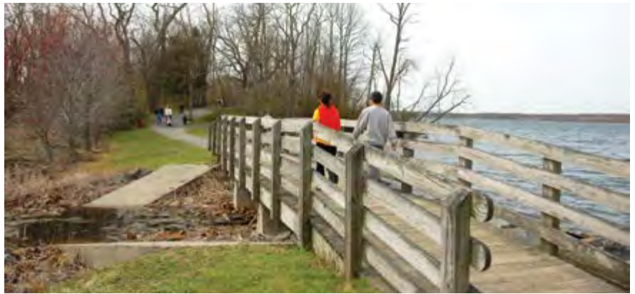
A bridge crossing over a wetland dike at the Manasquan Reservoir.
