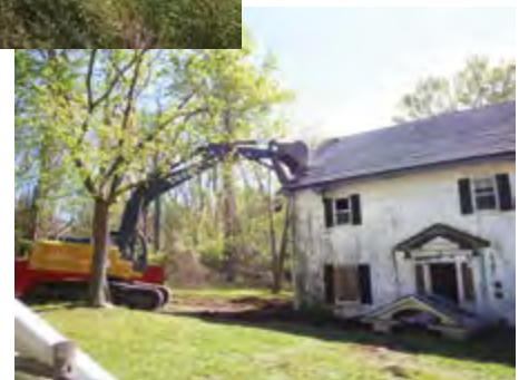
An old caretaker residence at Claypit Creek is cleared.
