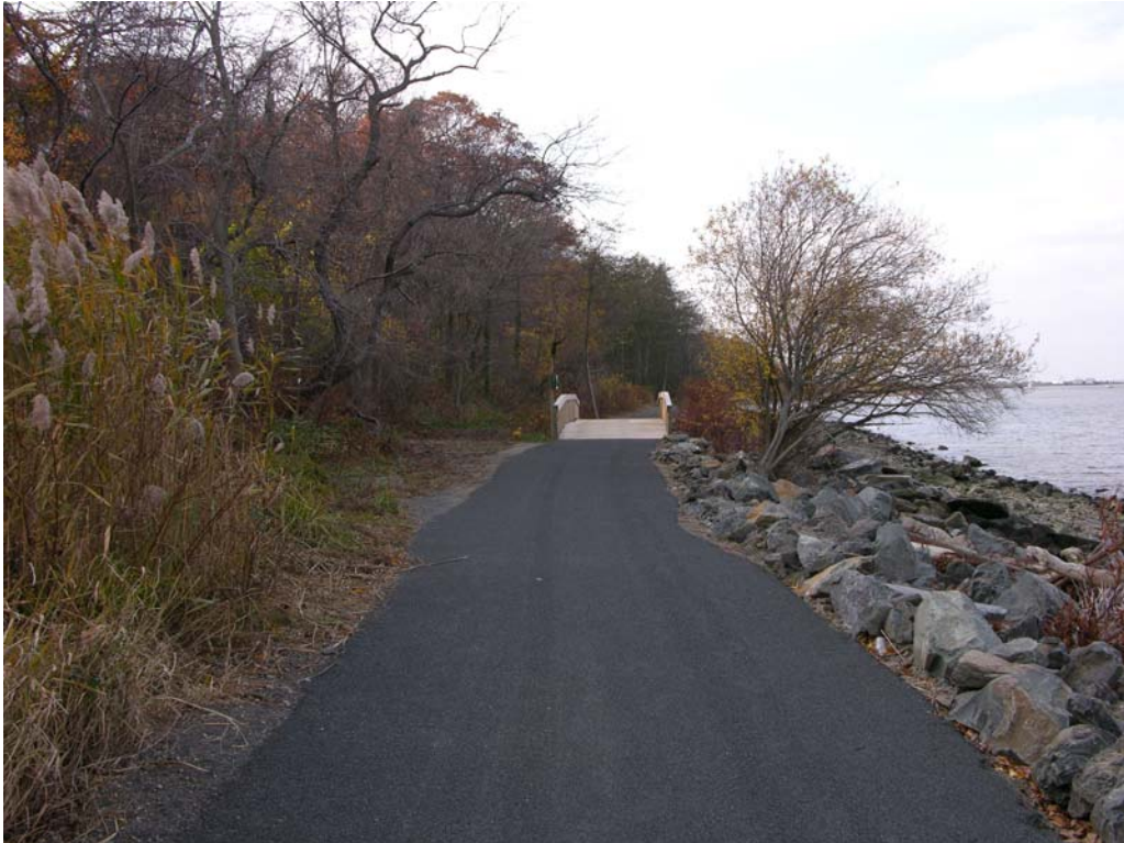
Henry Hudson Trail – Atlantic Highlands Trail and Henry Hudson Spring Bridge (Before Sandy)
