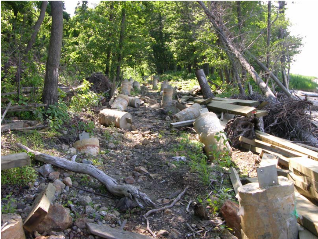
Henry Hudson Trail – Atlantic Highlands Long Bridge Section (Partial Cleanup, October 2013)
