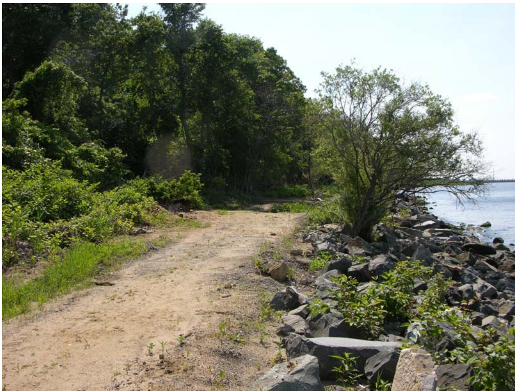
Henry Hudson Trail – Atlantic Highlands Trail and Former Location of Henry Hudson Spring Bridge (After Sandy, June 2013)
