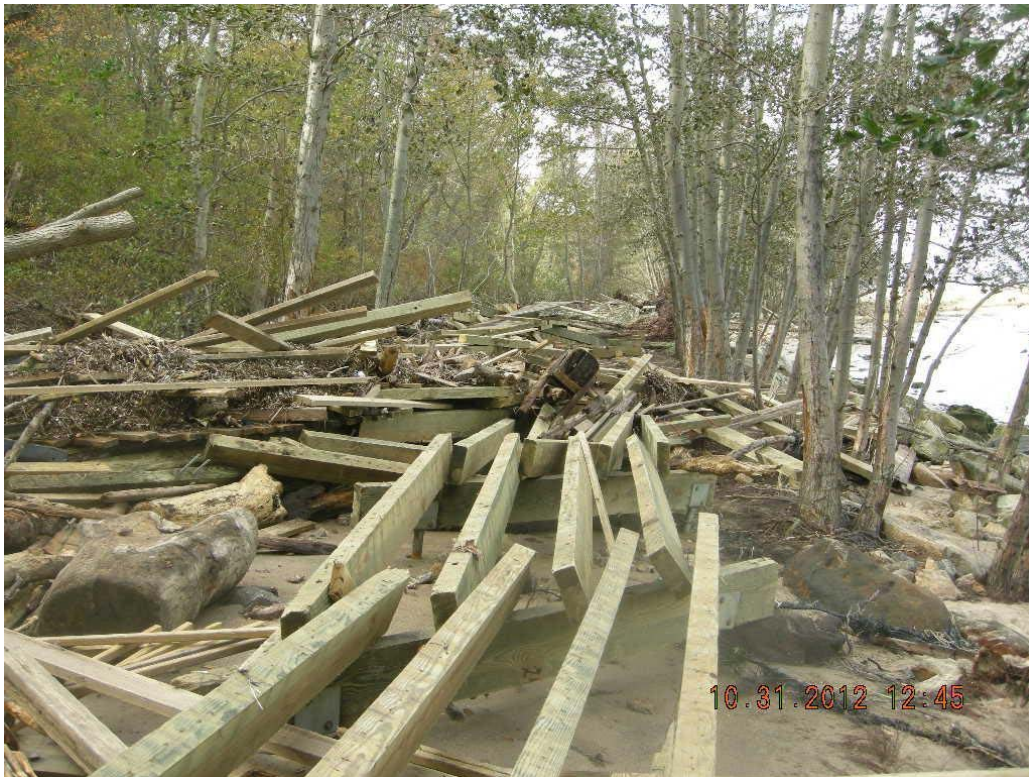
Henry Hudson Trail – Atlantic Highlands Long Bridge Section (After Sandy, October 2012)
