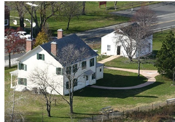
Bayshore Activity Center (left) and Activity Shed (right)
