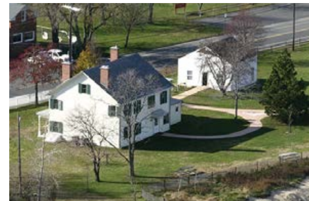
Bayshore Activity Center (left) and Activity Shed (right)
