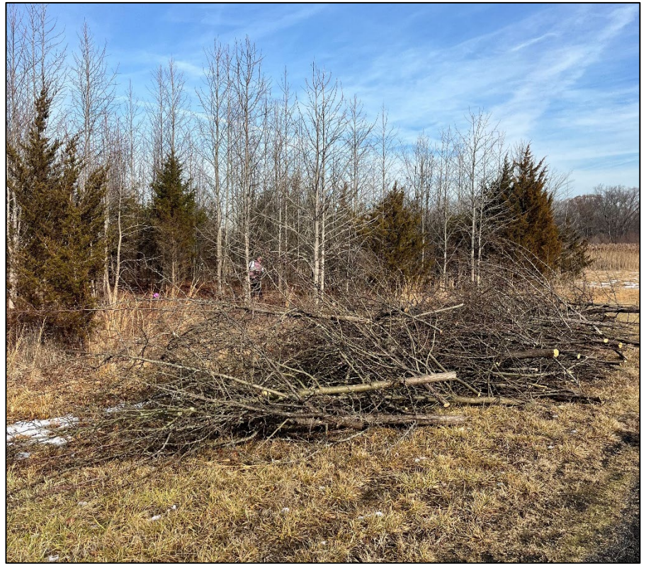
Invasive Callery pear removal near Track Edge trail.
