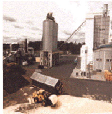
Built in Värnamo, Sweden, in 1993, the first plant to demonstrate the biomass integrated gasification combined cycle had a total efficiency of 82 to 83 percent and an electrical efficiency of 33 percent
